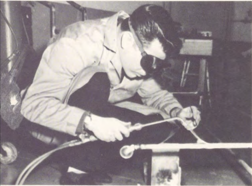
Using an acetylene torch, Mr. Canavit demonstrates the correct welding procedure to his industrial arts class.
